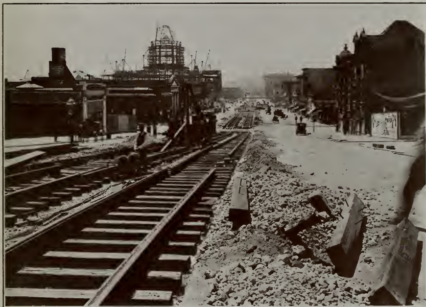
CONSTRUCTION OF VAN NESS AVENUE MUNICIPAL RAILWAY
